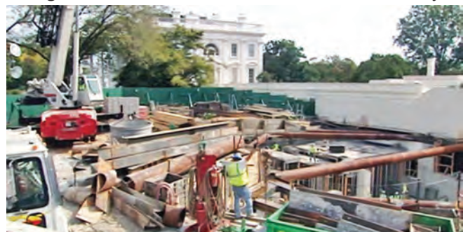
The 'bunker' under the north lawn under construction
